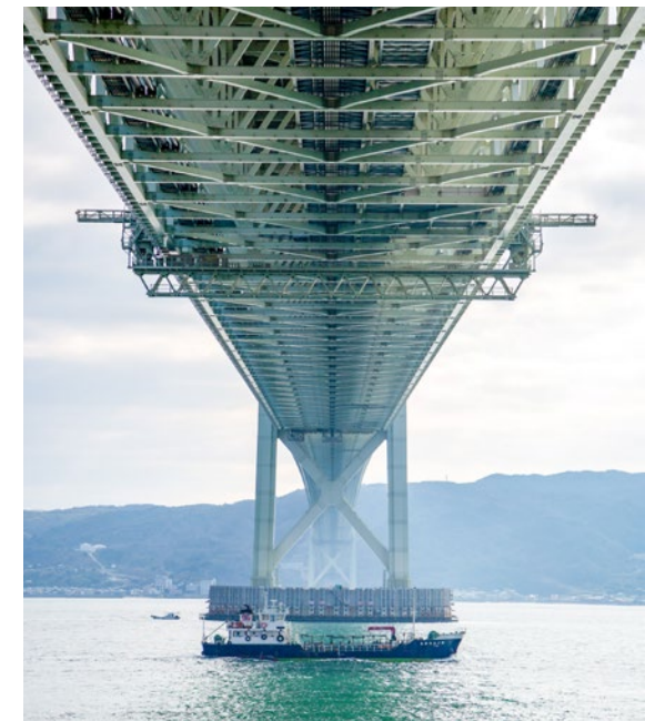
Under the Akashi Bridge Between Kobe and Awajishima
